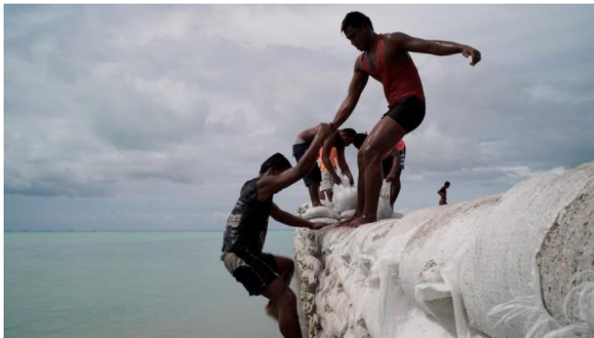
Young men build a wall of sandbags to protect against flooding in Kiribati, from Anote's Ark
